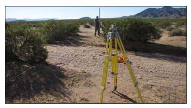
Figure 2.14: Measurements being taken using California rod and auto-level.
