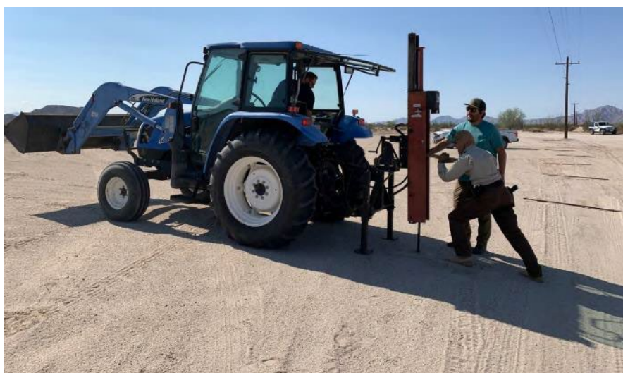
Road restoration work along 25E.
