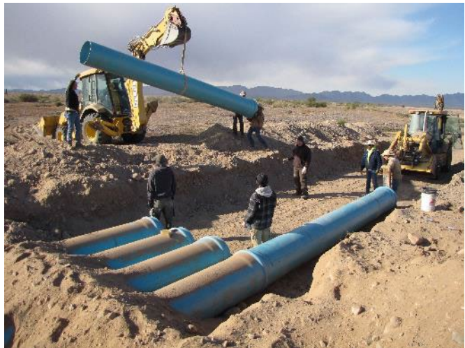
Barry M. Goldwater Range East staff construct a wildlife water in 2013.
