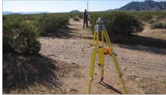
Measuring road elevation with a California rod and auto-level.
